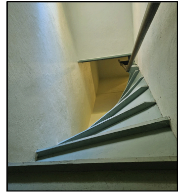
Back Staircase Used by staff, this staircase was also part of the Underground Railroad.
